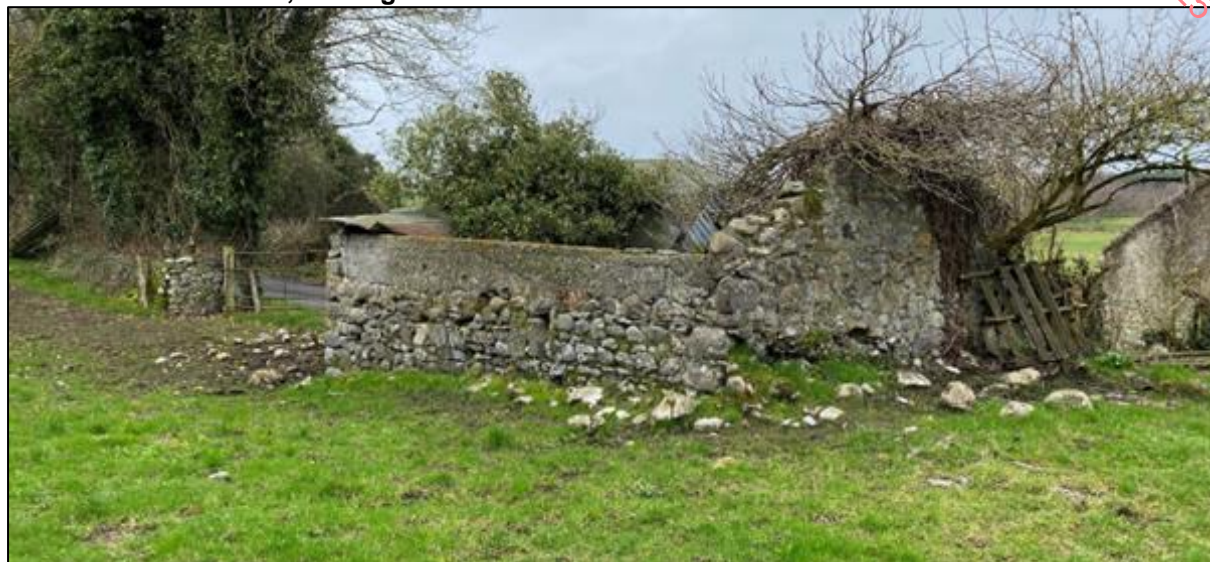
Plate 13-4: Structure 4, looking northwest
