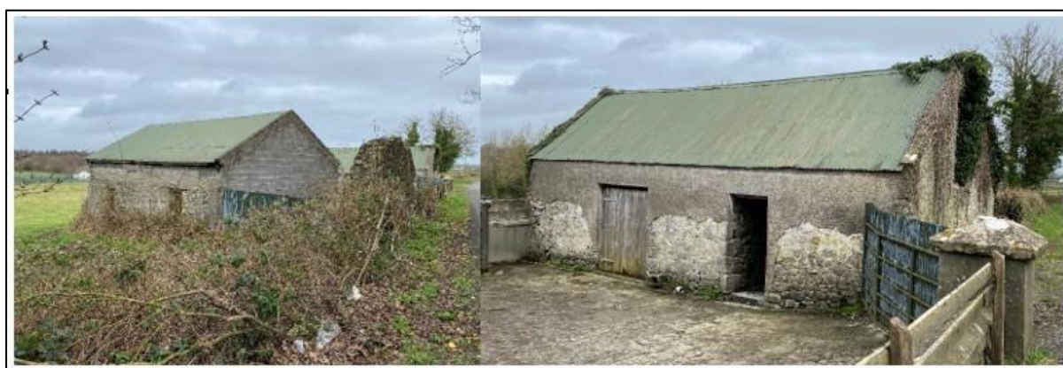
Plate 13-3: Structure 3, looking north
