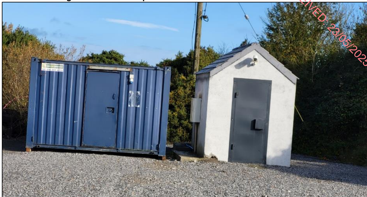
Plate 3-6: Existing Canteen and Pumphouse
