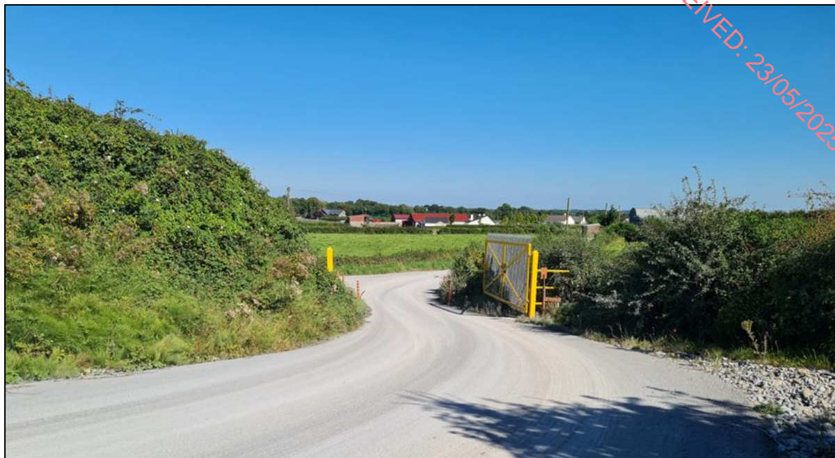
Plate 1-2: View of Access Road and Access Gate
