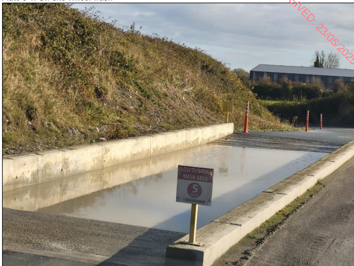
Plate 3-1: On-site Wheel wash
